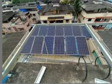
Commercial Solar Panel Installation Service
